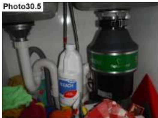
Waste disposer fitted and working.
