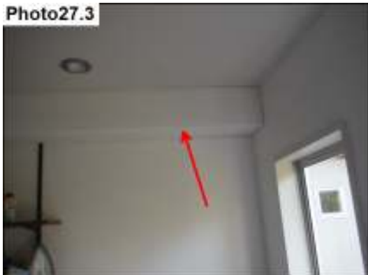
Duct from the toilet runs across the laundry area.
