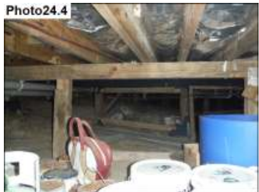
Silver foil is under the flooring. Drainage is well supported
