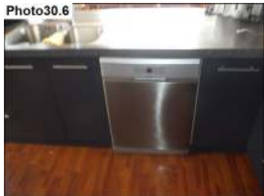
Dish washer fitted to the kitchen area.
