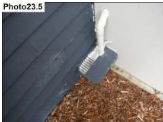
No smell or leaks noted to the gully traps.
