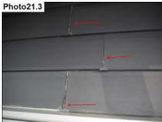
Back soakers fitted to the weather boards.
