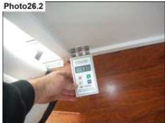
Moisture reading where scribe not installed. 13.0%
