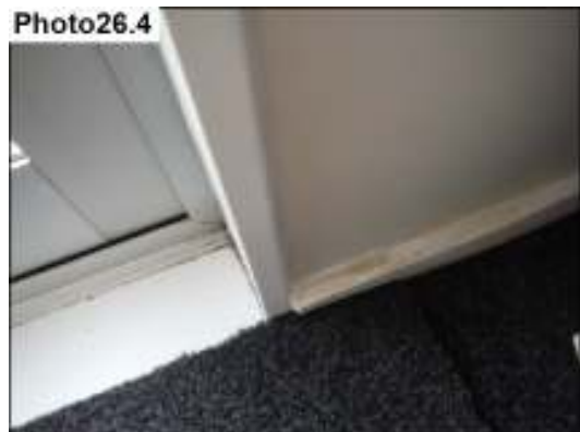
Repairs have been carried out to this ranch slider
