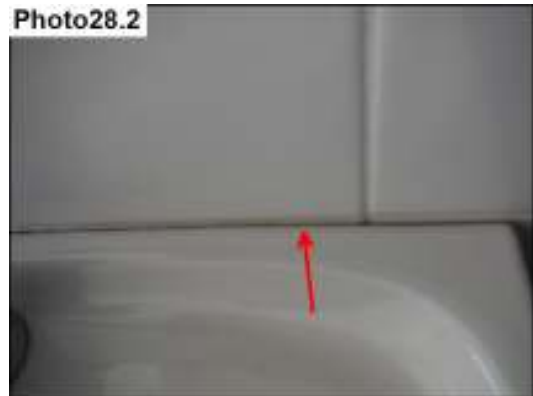
Photo28.2 Basins need to be silicone sealed against the wall.
